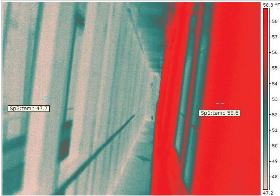
A. Thermal photograph of the solar wall at RiverEast
