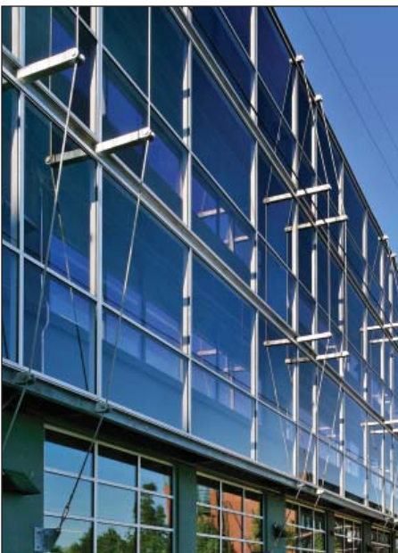
C. Solar wall constructed.
